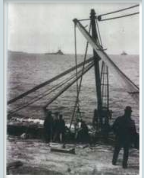
Repairing the pier, circa early 1900s. Image courtesy of Colin Scudls.
