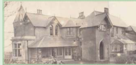
Ardfallen House, Dalkey, c. 1920. The Hollway family lived at Ardfallen before moving to Cabinteely in 1921. Anti-Treaty republicans unsuccessfully attempted to burn Ardfallen in October 1922 during the Civil War (Courtesy Philip Hollway).
