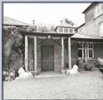
The front door at Fernhill, with rustic porch supported by wooden posts, c. 1990 (Courtesy Irish Architectural Archive).
