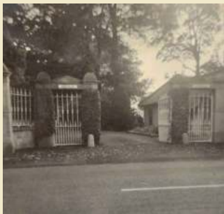
The gates and lodge to Airfield House, c. 1975 (Courtesy Irish Architectural Archive, Kevin Harrington Collection).
