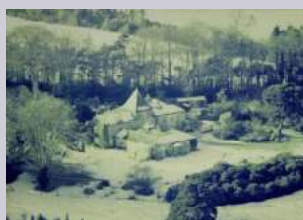
Aerial view of Fernhill House in the snow. The original building, constructed by Frederick Darley after he purchased the property, is visible with later additions behind it (Courtesy Nicholas Ryan).
