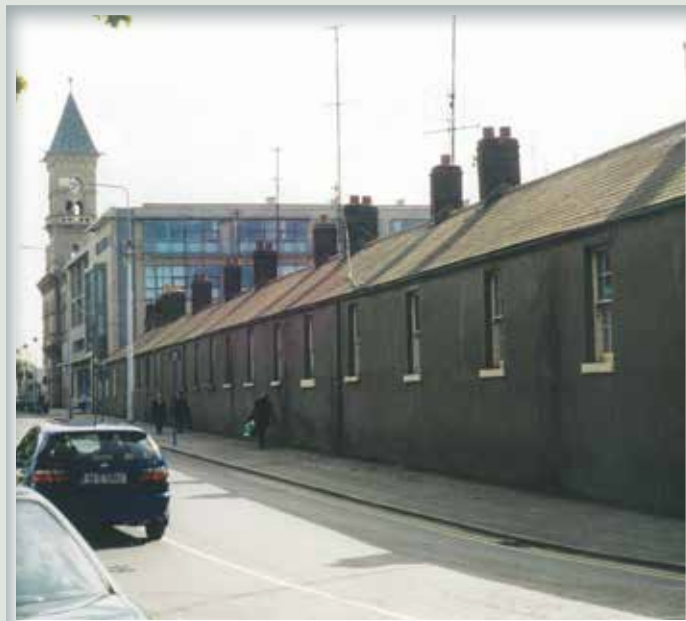
Harbour Commissioner's Cottages, Crofton Road, built 1820-40. Photo 2002. Demolished 2005. Image courtesy of Colin Scudds.
