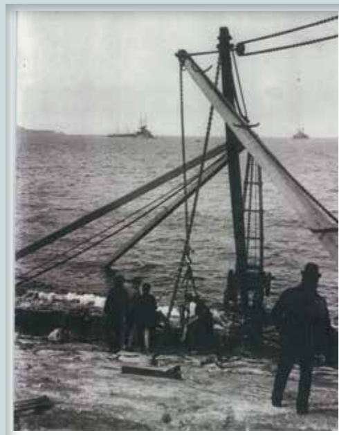
Repairing the pier, circa early 1900s. Image courtesy of Colin Scudls.
