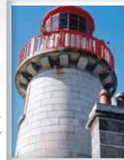
Detail of East Pier Lighthouse. 2012. Image courtesy of Colin Scudds.
