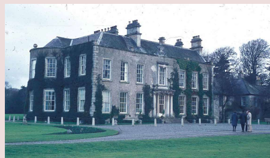
Marlay House, c. 1977. The house had been sold to Dublin County Council in 1972 and left empty. Comprehensive restoration work of the house would not begin until 1992 (Courtesy South Dublin Libraries, Patrick Hely Collection).
