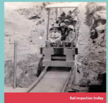
Rail inspection trolley
