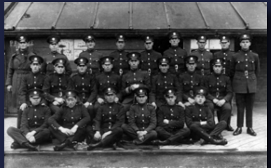
Defence Unit, McKee Barracks extension to Phoenix Park Depot 1923
